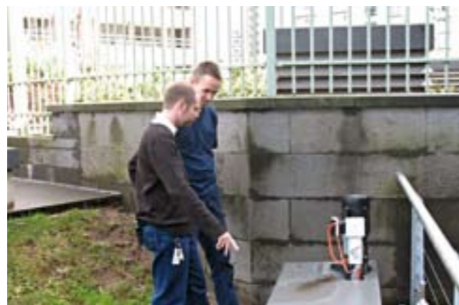
Mike Cardiff, Facilities Operations Co-ordinator and Aaron Grigg of Honeywell, inspecting NGV International moat water recycling systems
